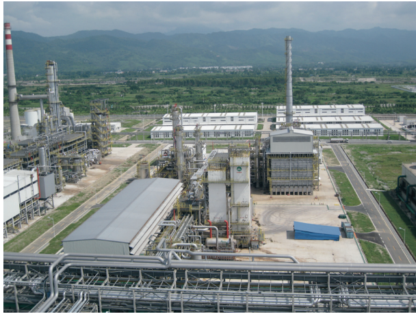
Figure 1. Air Products and PetroChina recently brought onstream a steam methane reformer (SMR) that produces over 90 million ft 3 /d of hydrogen and syngas to support PetroChina's Sichuan refinery and petrochemical facilities.
