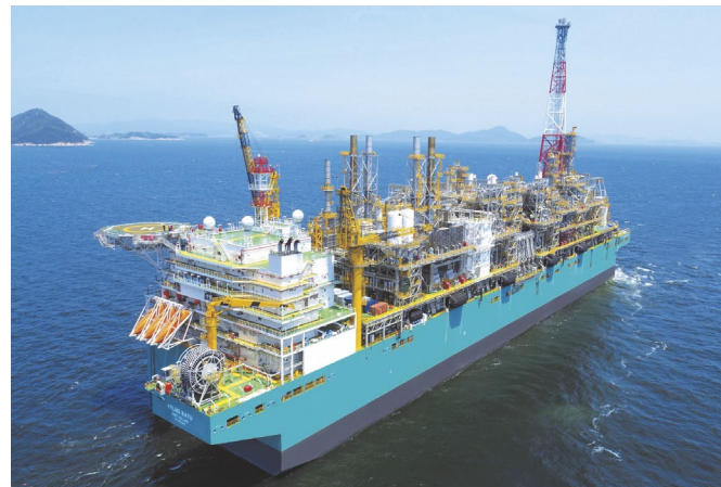
Petronas FLNG Satu, Malaysia utilizes Air Products' Nitrogen (AP-N™) LNG Process (Photo courtesy of Petronas)
